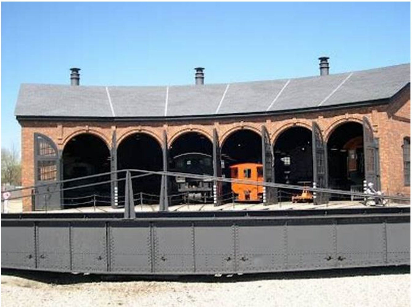
A steam locomotive undergoing maintenance inside the roundhouse of the Detroit, Toledo & Milwaukee Railroad in Flat Rock, Michigan.
